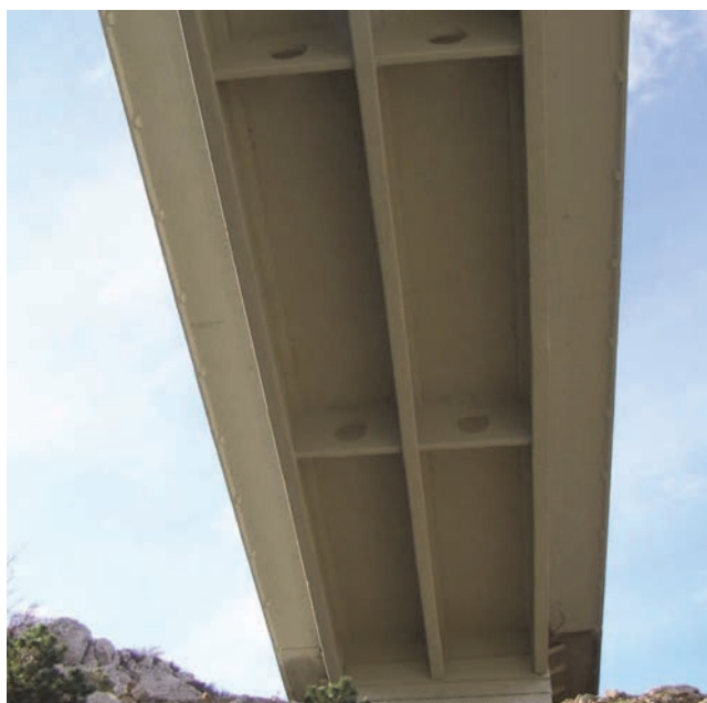
Figure 15. Deck slab bottom contour in the U5-S31 zone after application of the final coat of paint [14]
