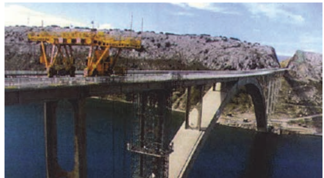
Figure 7. Load relieving scaffold at pier S26 [4]
